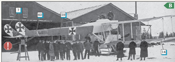
Gotha G.1 11/15. Note where the original serial number has been overpainted, the modified cockpit coaming with cupola gun ring and tail skid trestle.
